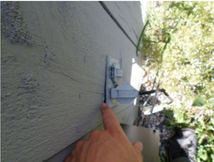
Observed the exterior Garage electrical outlet to be very loose, Also did not appear to be GFCI as required in today's standards. Contact a licensed electrician to make the necessary repairs
