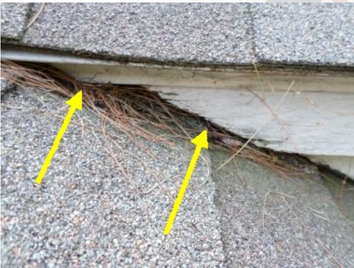
Wood rot observed. Wooden trim adjacent to the roof surface should have at least an inch of clearance from the roof covering (and more in snowfall areas) This leads to the wood wicking the water and rot.
