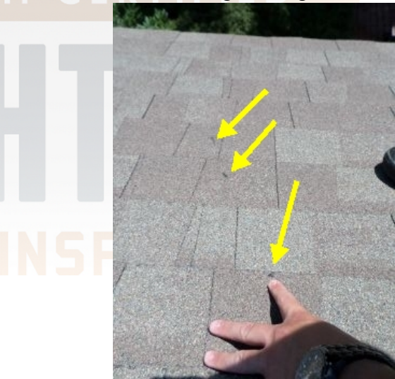
Note: Roof covering damage was observed.
