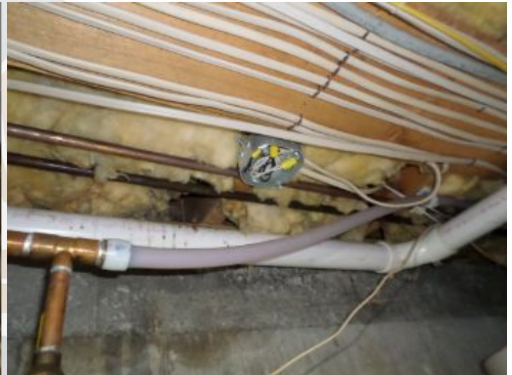
Observed an open junction box under the crawlspace area. For safety reasons have a new cover installed over the box.
