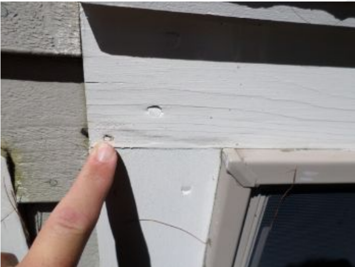
Wood rot noted. Recommend contacting a qualified general contractor to make necessary repairs.
