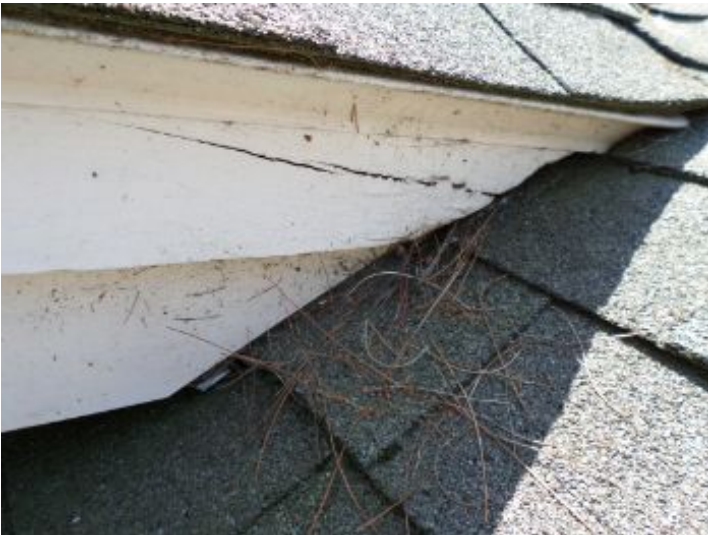
Wood rot noted. Recommend contacting a qualified general contractor to make necessary repairs.
