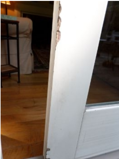
Note: Door damage on siding door.
