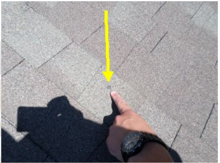
Note: Roof covering damage was observed.
