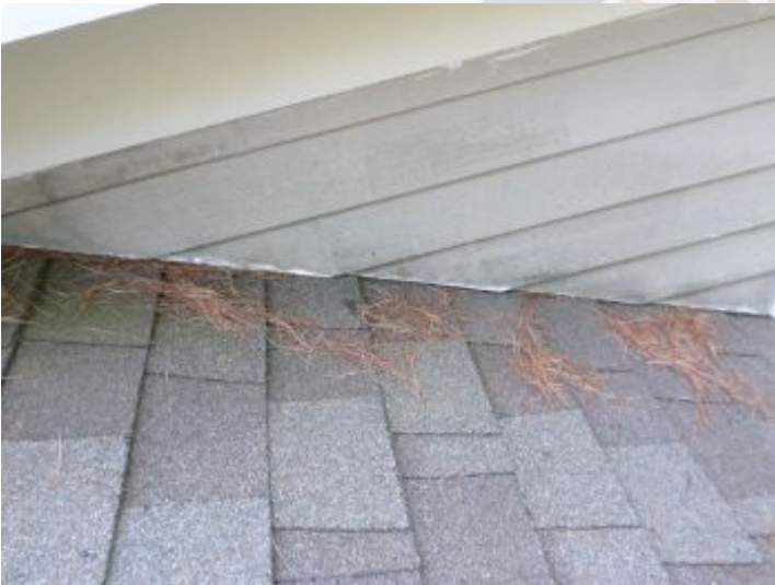
Observed that the siding was too close to the roof covering. Wooden siding adjacent to the roof surface should have at least an inch of clearance from the roof covering (and more in snowfall areas)
