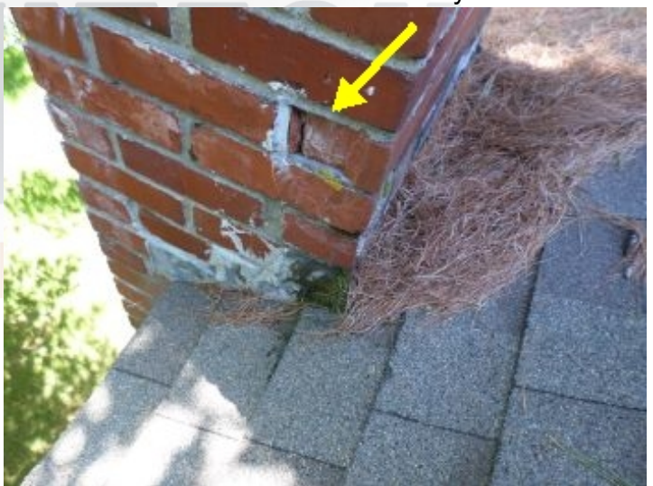
Note: Spalling was observed.
