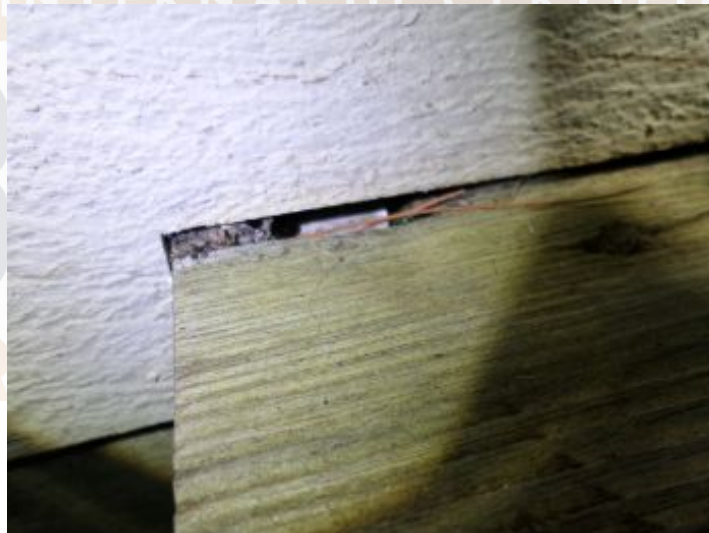
Note: It appeared that there is no flashing installed the deck Ledger attachment to the structure.
