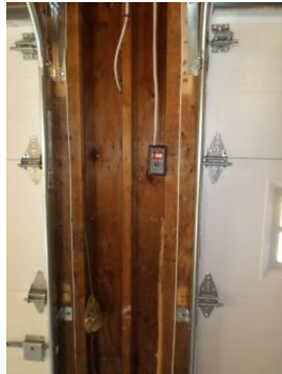
(Safety concerns) , consider installing a GFCI outlet in the garage, as this is today's standards for safety.
