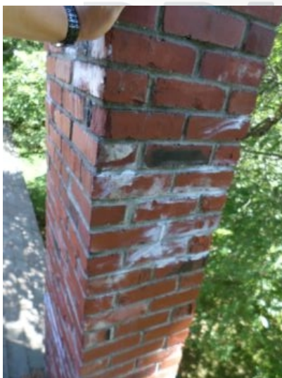
Observed what appeared to be some sort of silicone caulking smeared into the mortar joints.
