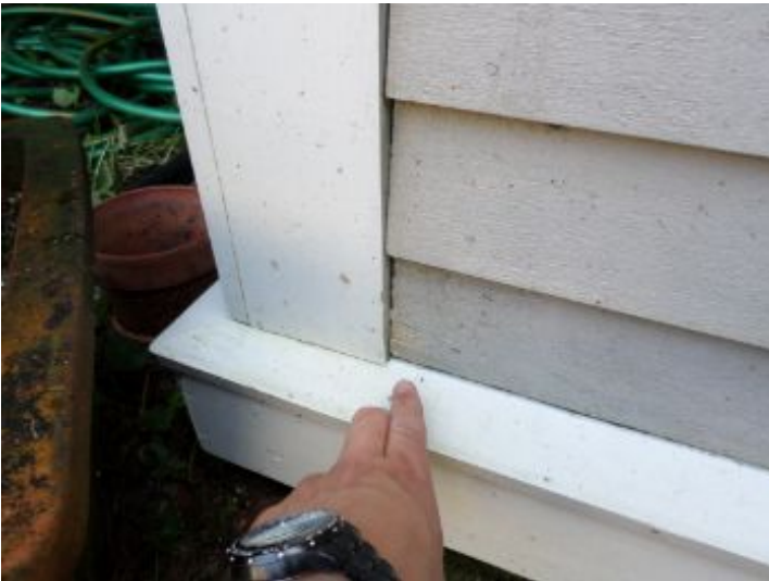
Softening wood was observed.
