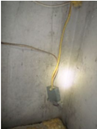
Observed in unsecure junction box under the crawlspace area. Recommend affixing it to the proper location
