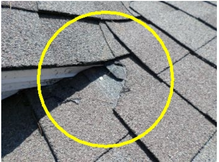
Observed damage to the roof covering. This may be caused by an uplift from the wind. Recommend contacting a qualified roofing contractor to make necessary repairs.
