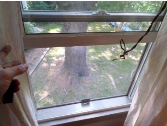
Egress bedroom window was operable at the time the inspection
