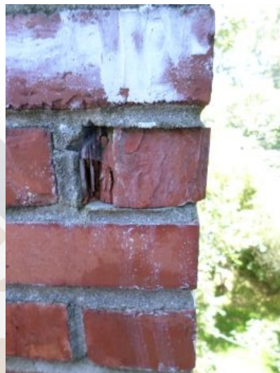
Observed deterioration (spalling) of the bricks on the Southside chimney.
