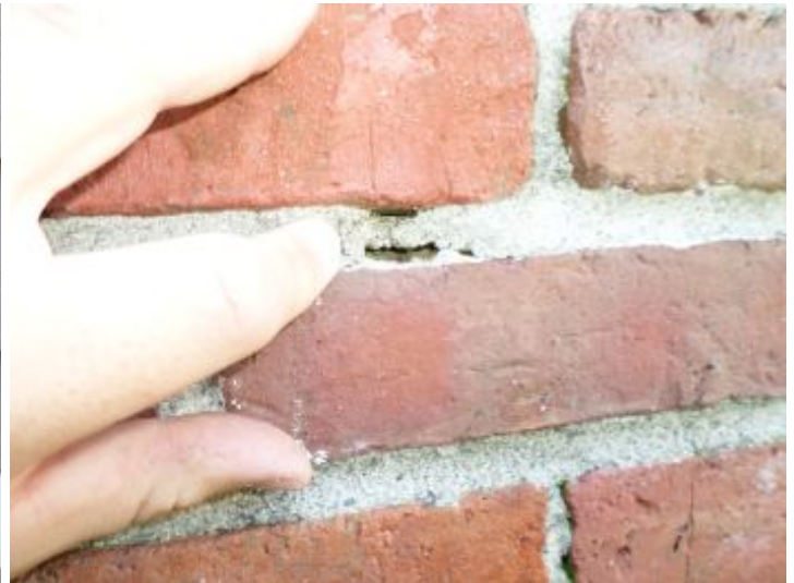
Repointing of the bricks would be recommended in the next few years.
