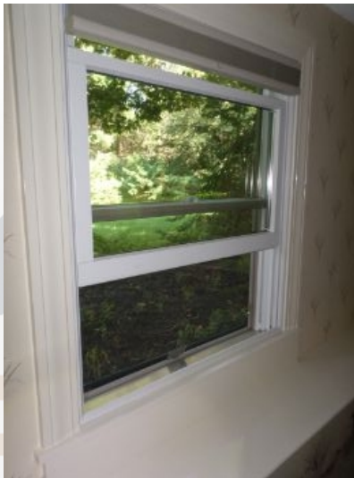
Egress bedroom window was operable at the time the inspection
