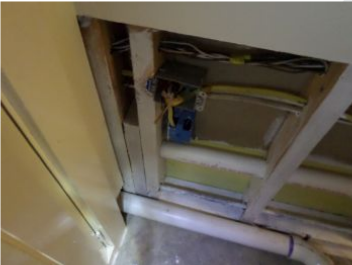
(Safety concern) observed in open junction box in the utility closet. Contact a licensed electrician to make the necessary repairs
