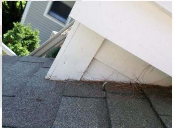
Note: Siding was too close to roof coving.
