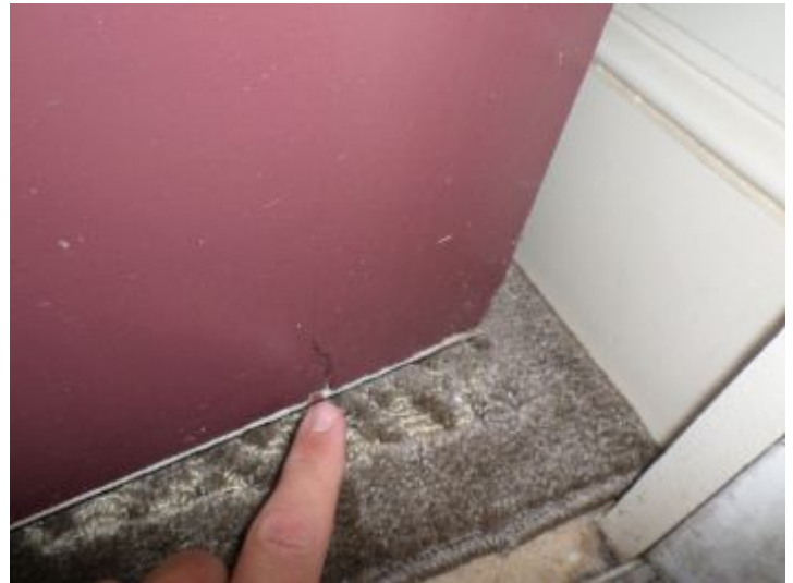
Wood rot was observed at the bottom of the front exterior door. Consider budgeting in upgrading the exterior doors. Also, once consider installing a storm door to help with heating/cooling costs
