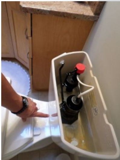
The top tank on the toilet was a bit loose, re-tighten is necessary
