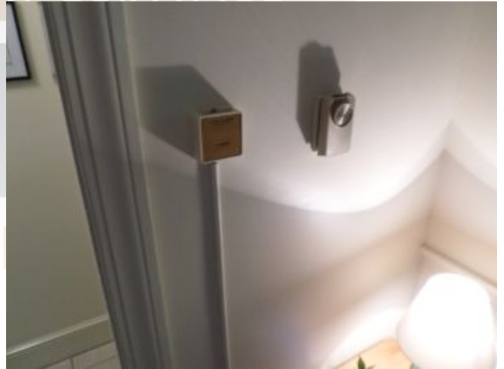
Gas stove thermostat.
