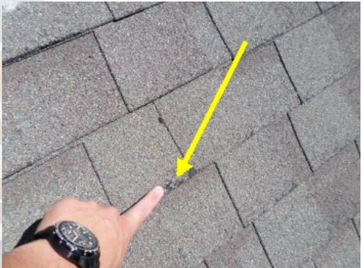
Observed damage to the roof covering. This may be caused by an uplift from the wind. Recommend contacting a qualified roofing contractor to make necessary repairs.
