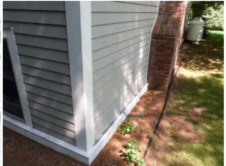
Observed wood trim in contact with the ground. This will lead to premature wood rot, due to moisture wicking. Contact a qualified contractor to make necessary repairs. Please see graphic
