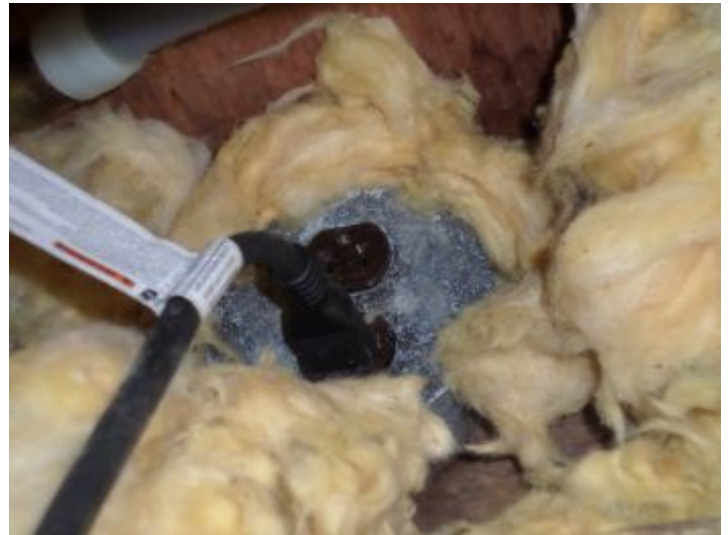
Observed the outlet that supplies energy for the sump pump is not a GFCI. This is a safety concern, since it has direct access to water.
