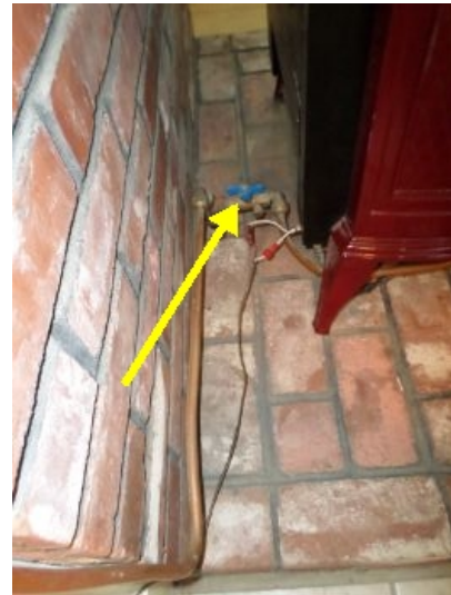
Gas Stove shut off.
